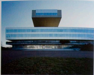
Foto Photo Pez Hejduk, 2011 Architektur Architecture Georg Lippert Projekt Project AUA – ehemalige Firmenzentrale der former headquarters of Austrian Airlines, Wien (AT), 1978, Abriss Demolition 2013
